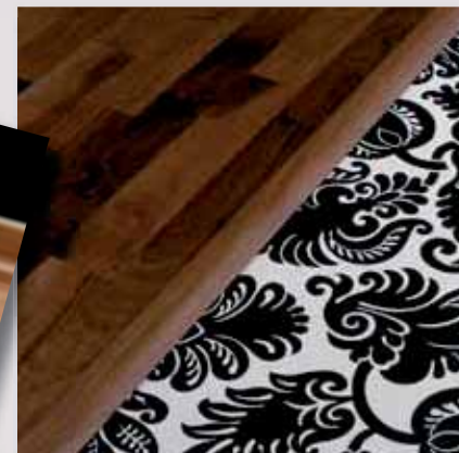
The reducer is used to smooth the transition.
